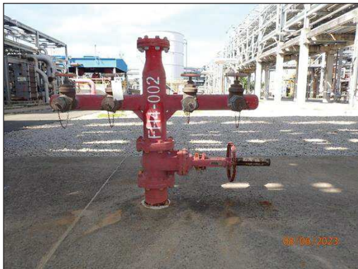
Fire Hydrant/Monitor
